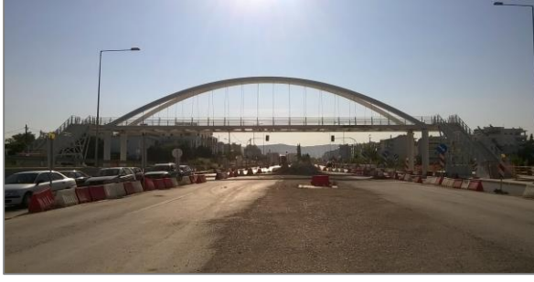
Fig. 2. The pedestrian bridge in Evosmos, Greece
