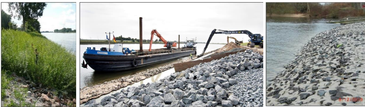
Figure 1: Different types of bank protections at inland waterways: technical-biological bank revetments, riprap revetments and grouted armour stone revetments (Photos: BAWArchiv)
