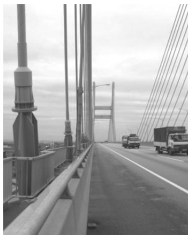
*Fig.5.2 Accessibility to cables of cable-supported bridges-Starossek (2008)*
