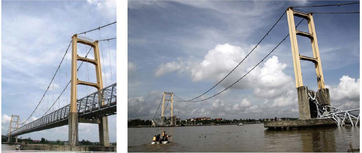
*Fig. 2.5 Mahakam II Bridge in Indonesia before and after the collapse (Qiu et al. 2014)*
