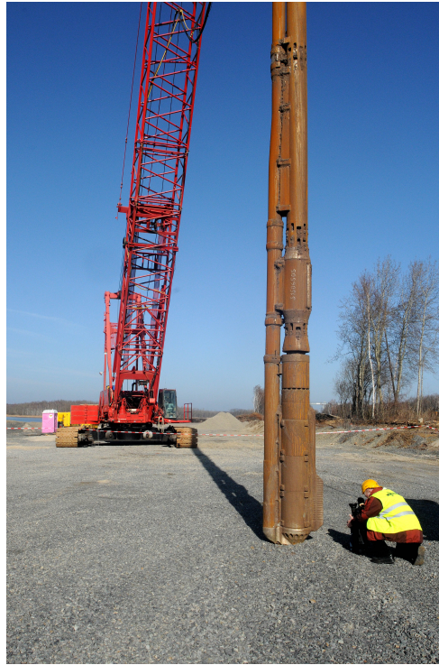
Figure 1.2: Deep vibration compaction probe at work in Silbersee, North Germany
