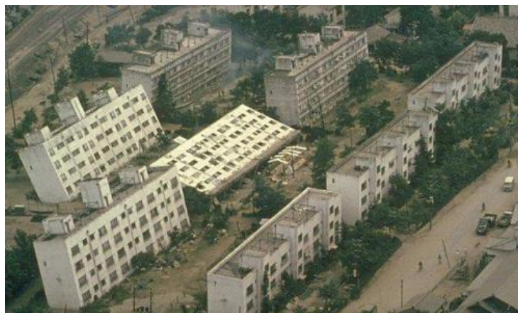
Figure 1.1: Liquefaction induced damage in the 1964 Niigata, Japan Earthquake (Elnashai and Di Sarno, 2008)
