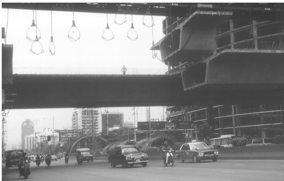
Abb. 3.1: Segmentbrücke des “Second Stage Expressway” in Bangkok
