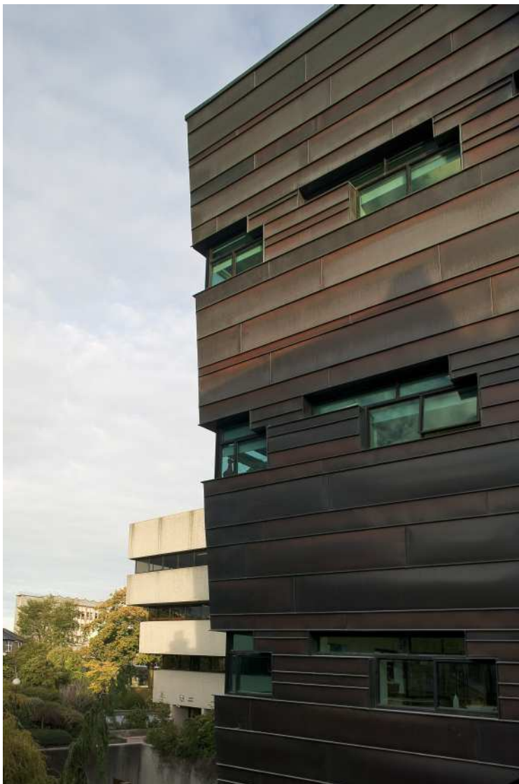
Oxidised Copper for the facade (Photo: Wilson Architecture)
