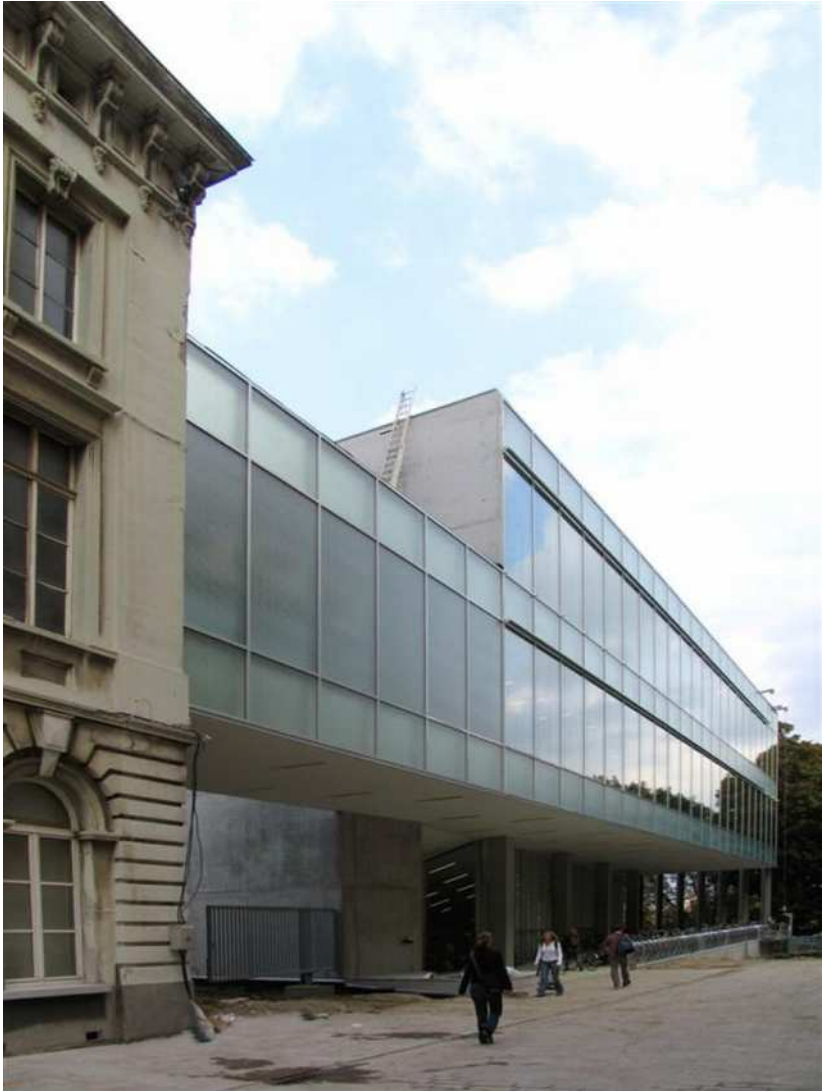
Facade and entrance (Photo: Beel architects)
