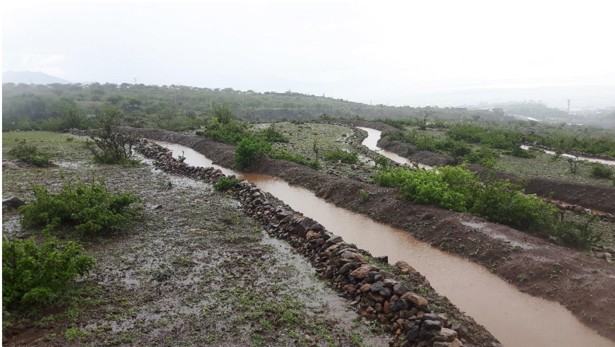
Figure 27: Contour line trenches retaining water during a rain event in the Slope Farming Project site, Arba Minch, Ethiopia. Wibbing (2017).
