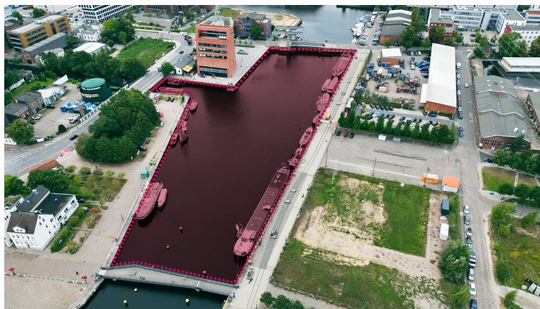
Figure 5: The Lotsekanal (Pilot's Channel), situated in the Port of Hamburg, has been chosen for conducting the sea trials. The designed area, marked with dark-red colour, is approximately 200 m long and 65 m wide in its broadest point
