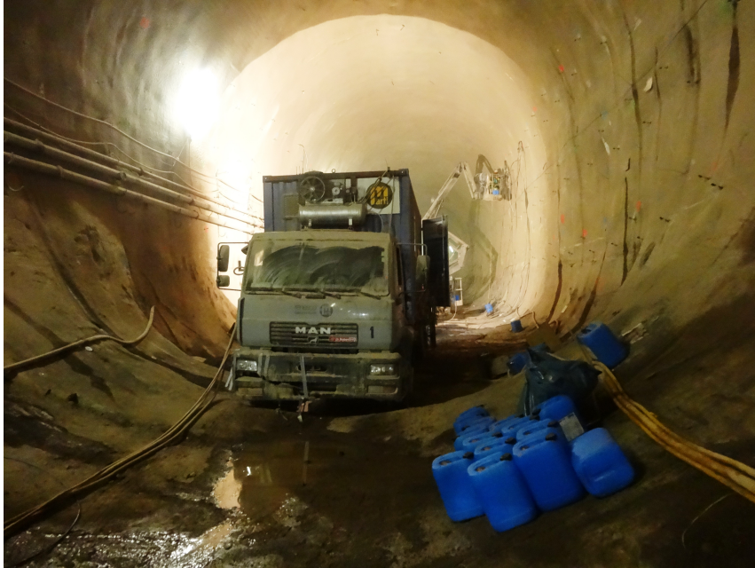
Figure 7.8: GEA, an AC injection unit. Visible are the truck and the container mounted on the truck. One of the two chemical components are stored in blue canisters and visible in the bottom right of the picture. In the background one of the lifting platforms raises to allow a worker the access to a borehole in the upper part of the tunnel.
