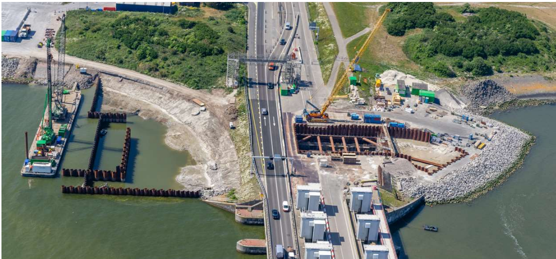
Figure 1: Top view of one of the construction phases on site
