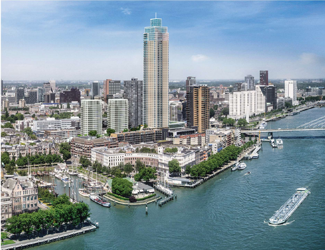
Figure 1: Zalmhaven tower, Rotterdam (after Schippers et al., 2021)
