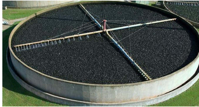
Figure 26. Conventional trickling filter (Greenion, 2014)
