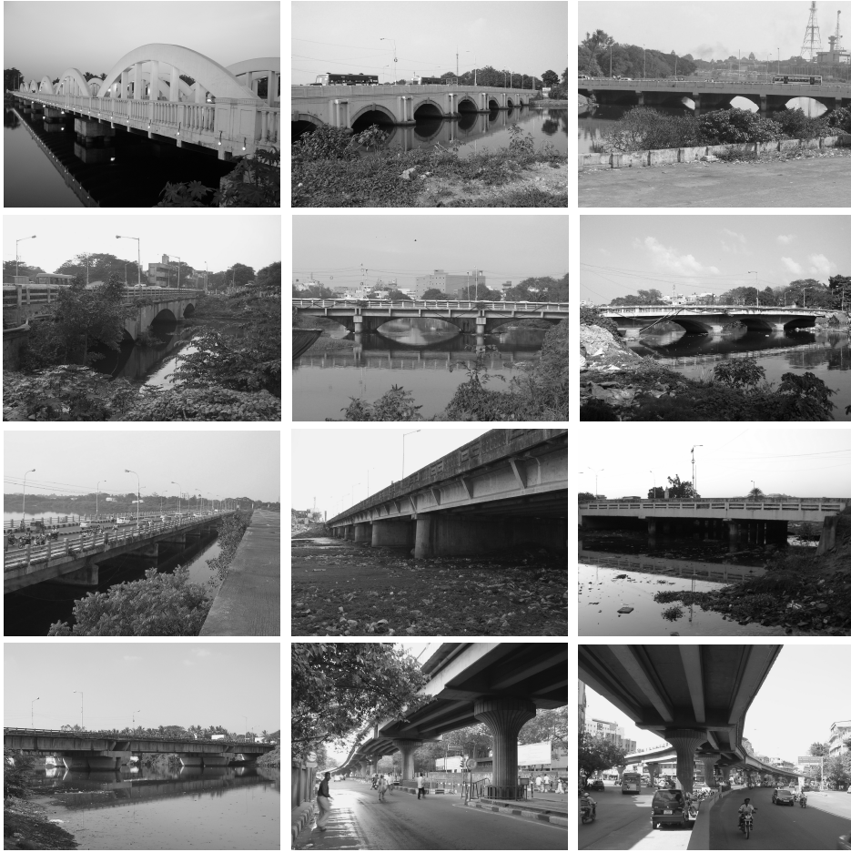
Fig. 3.4: Chennai Bridges (from left to right): First row: Napier Bridge, Periyar Bridge (from west, historic bridge), Periyar Bridge (from east, broadened with reinforced concrete girders); Second row: Harris Bridge (from north, historic bridge), Harris Bridge (from south, broadened with reinforced concrete girders), St Andrew Bridge; Third row: Thiru Vi Ka Bridge, Maraimalai Adigal Bridge, Quaid-E-Millet Bridge. Fourth row: Kotturpuram Bridge, Sardar Patel Rd Flyover, Adyar Flyover (Photos: Grischa Dette)
