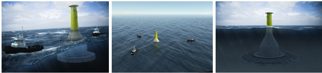
Figure 1.1: Towing, stabilizing and installation of gravity foundations (Source: Seatower AS).
