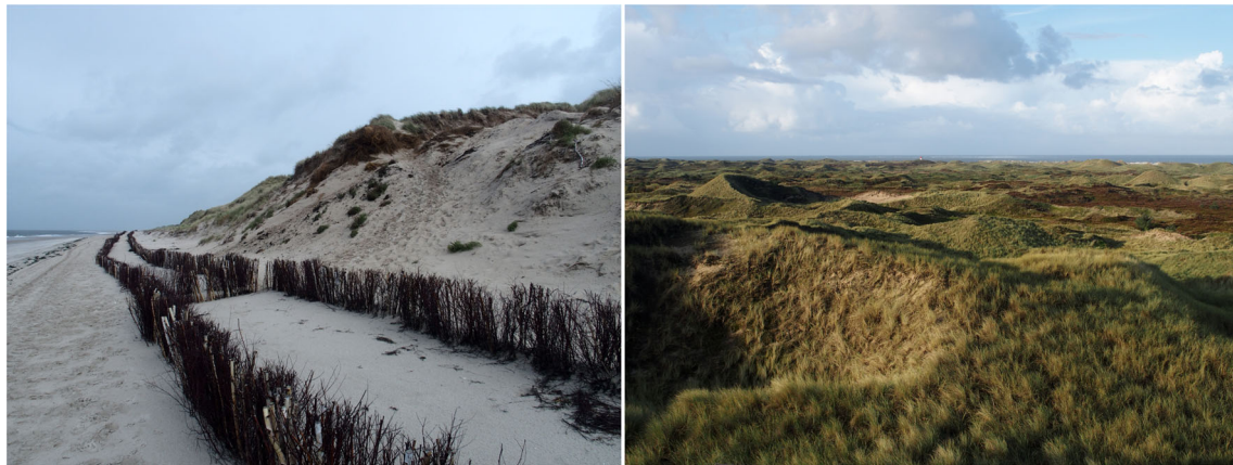
Fig. 9 Bush fences in front of the dunes to accrete sand at Amrum Odde (left) and vast dune area near Norddorf (right), Photos: P. Jordan
