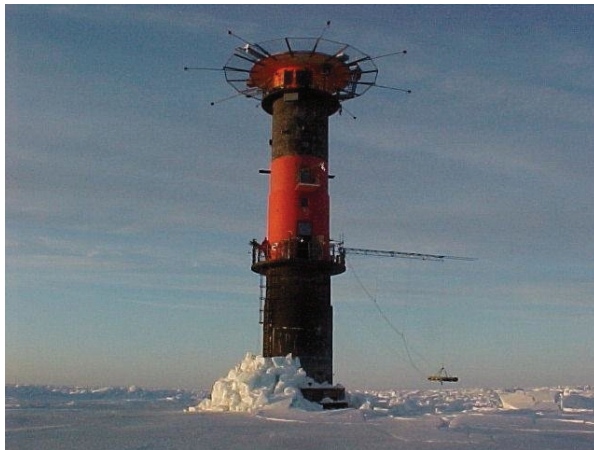
Figure 4: Photograph of Norströmsgrund Lighthouse with rubble accumulation after crushing failure of drifting level ice (Photo by Kari Kolari, VTT)
