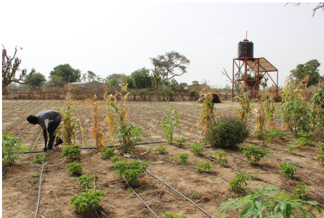
Figure 3 A Solar-Powered Pump System Is Combined with Drip Irrigation at Faylar Village in Senegal
