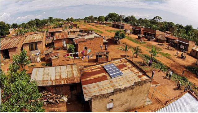
Figure 5 The 500 W Solar System Powers a Home, a Public Broadcasting System, a Barbershop and a Video Hall in a Rural Village in Uganda
