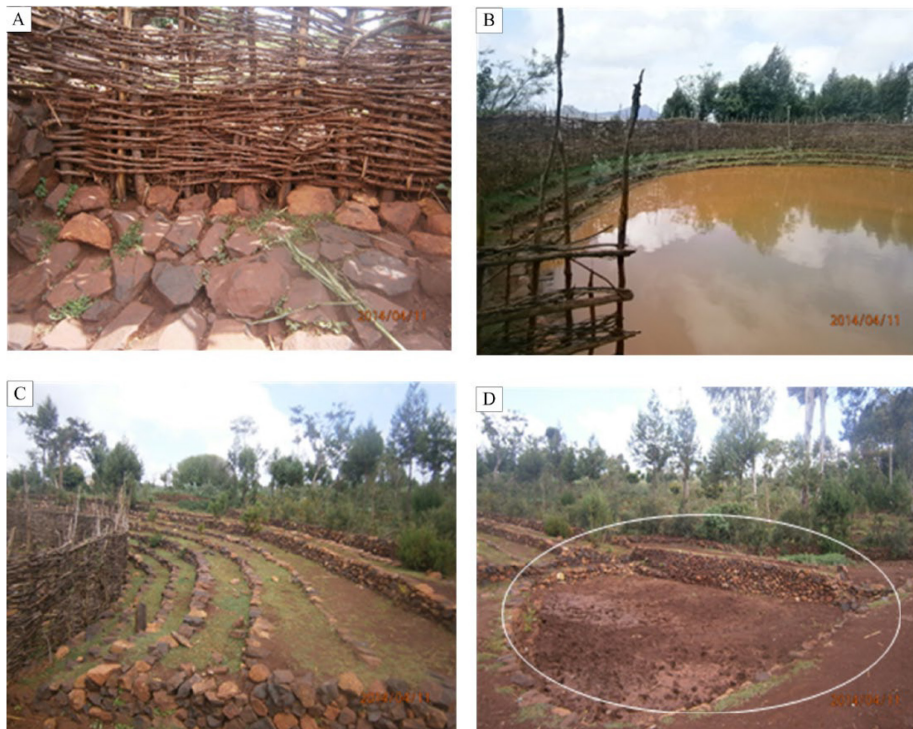
Figure 2 (a) A Wooden Mesh to Sieve Debris, (b) Fenced Pond, (c) Preserving Ponds from Silt by Constructing Outside Terraces, and (d) Basins to Collect Silt Coming in through the Flood (Behailu, Pietilä & Katko 2016, p. 8)
